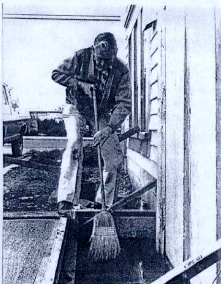
TOM MCIVER takes steps for safety at the Qualicum Beach and District Cultural Centre by roughing up wet cement with a broom. When the cement dries, the grooves will make the steps rough, preventing slippage in wet, cold weather. McIver and other volunteers are nearly done restoring Qualicum's Old School into an art centre and gallery where local artists will work and teach. The centre may be finished by Christmas.
